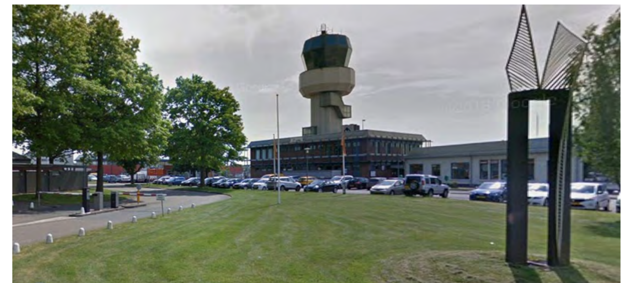
4. Parkeerterrein zone vertrekhal (Bron: Google maps).
